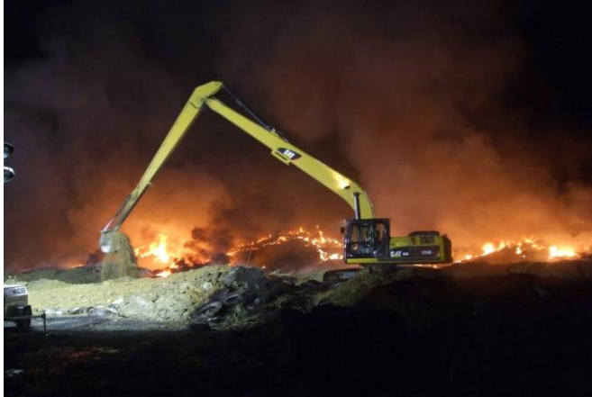
The contractor placed soil over the tire fire at King Tire Recycling in an effort to extinguish the fire. (EEC Photograph)
