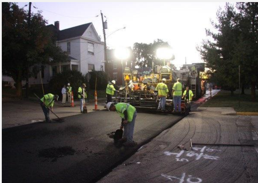
Eaton paving train applying rubber modified asphalt in Dayton, Ky., near the Ohio River. Photo by Mark Belshe, Rubber Pavement Association (RPA).
