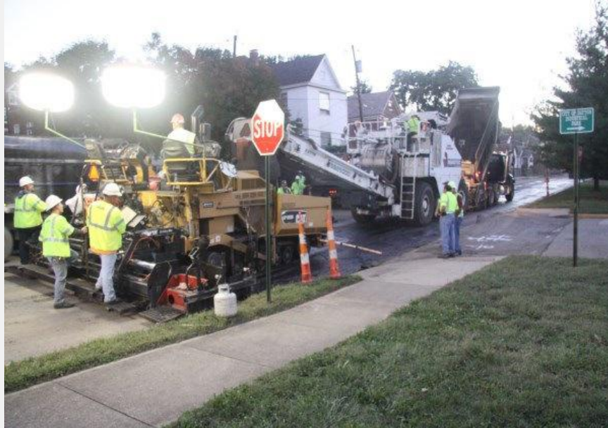
Eaton paving train applying rubber modified asphalt in Dayton, Ky., near the Ohio River. Photo by Mark Belshe, Rubber Pavement Association (RPA).
